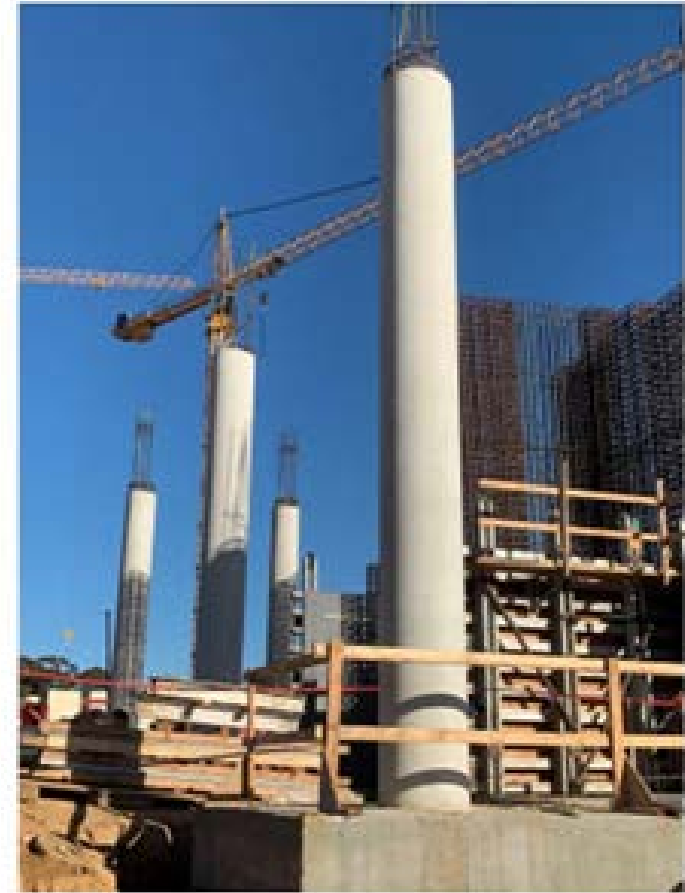
PLC Concrete at UCSD
