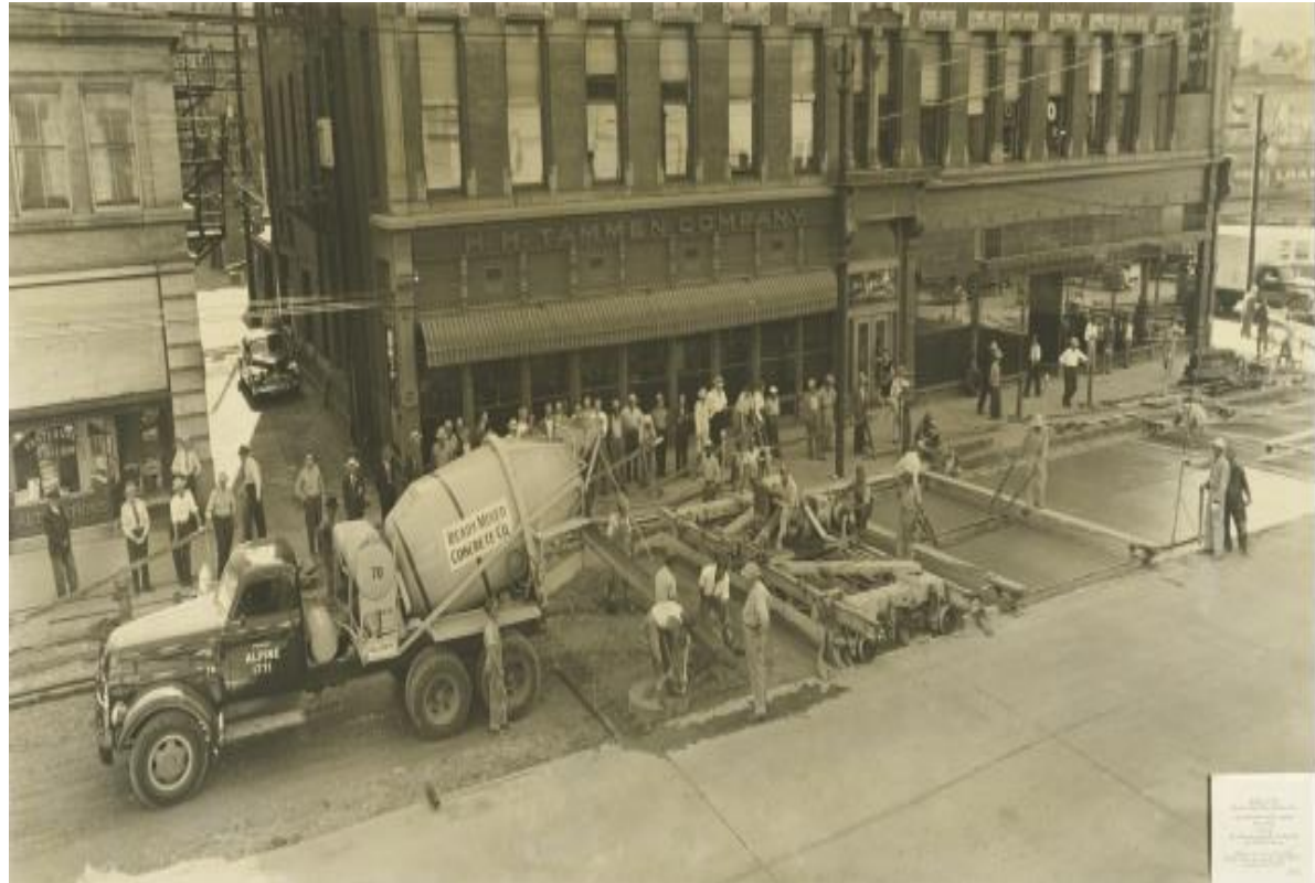
Ready Mixed Concrete placing concrete along 17th Avenue in Downtown Denver, early 1950s
