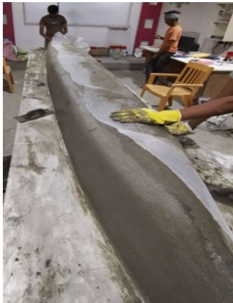
Figure 13: Mesh Overlapping
